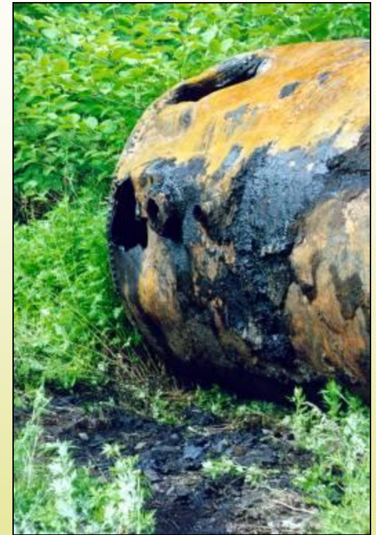
UST removal at Riverside Hills, Providence, Rhode Island
